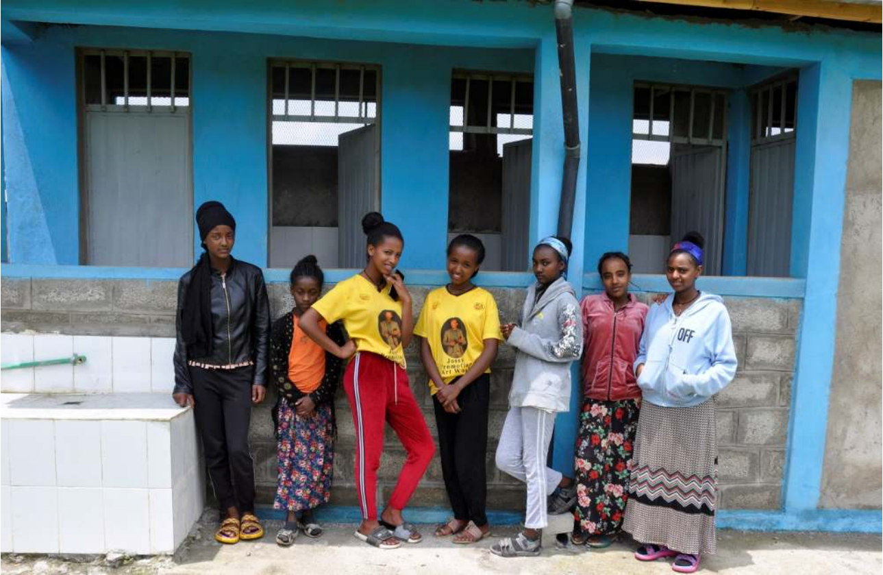
Meaza (1 st from right), Kalkidan (2 nd from right) and other girls at newly constructed toilet and hand-washing facility
