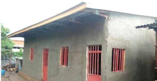
Nearly completed house for leprosy affected family in Ambo town
