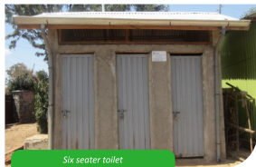
Six seater toilet
