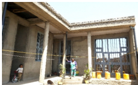
Recently completed house through self-help saving group scheme
