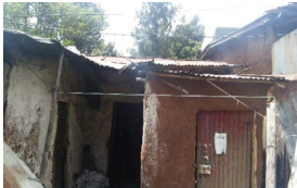
A house before renovation
