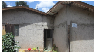
A house after full renovation
